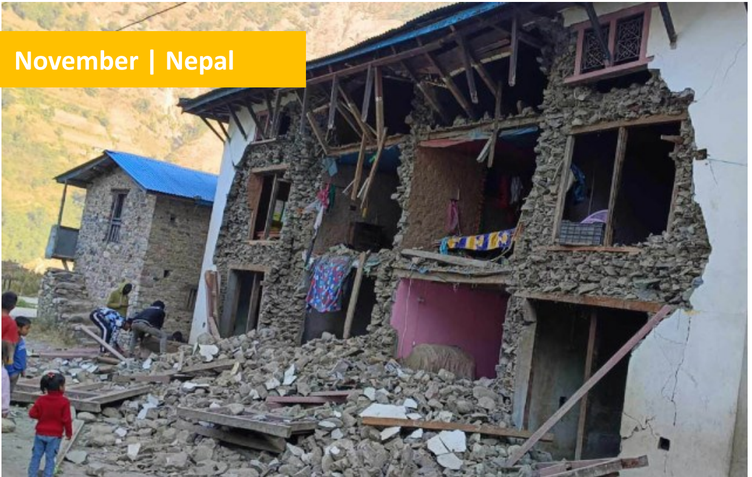
Source: The Kathmandu Post ( full article ) A house in Aathbiskot Municipality-12 of West Rukum damaged by the quake. Photo:
