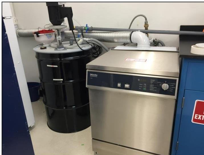
**Figure 46. Miele G7899 washer-disinfector with wastewater decontamination system.**
